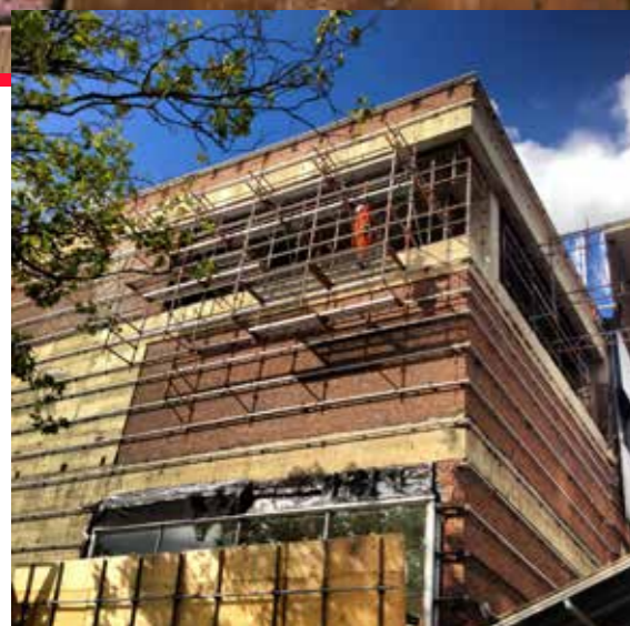
Project in de steigers
