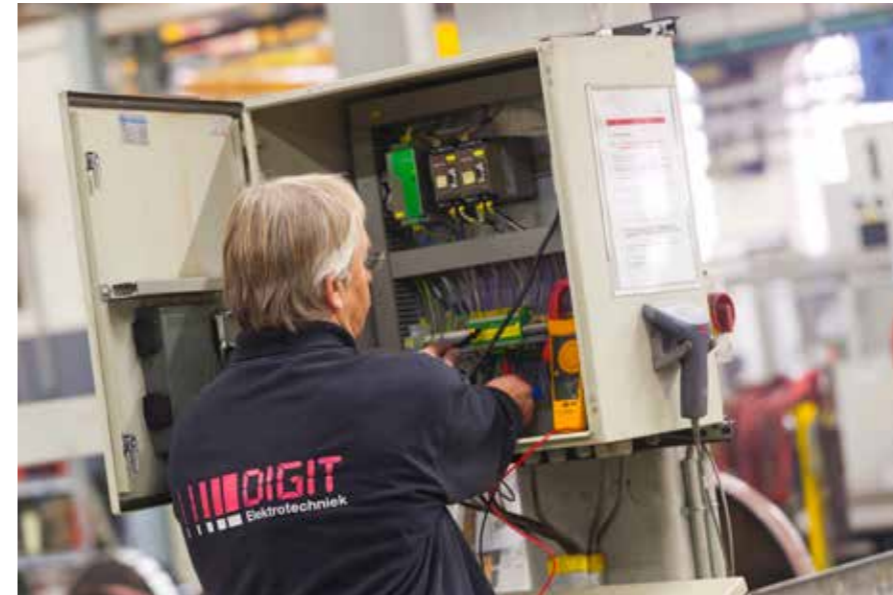
Metingen in schakelkast
